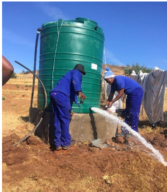
Water monitors connecting pipes from the tap to the tank for community members to collect. Photo credit: Mzingisi Nyhodo, CSA
