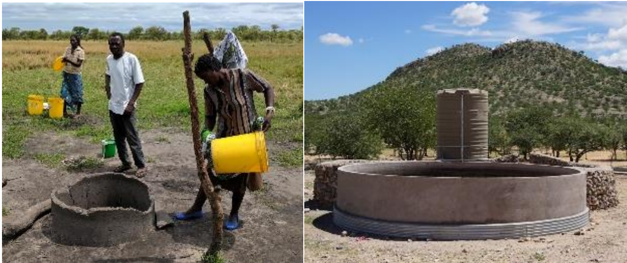
Construction of wells and water tanks help communities maintain water supplies in times of drought, Kenya. Photo credit: Nikhil Advani, WWF
